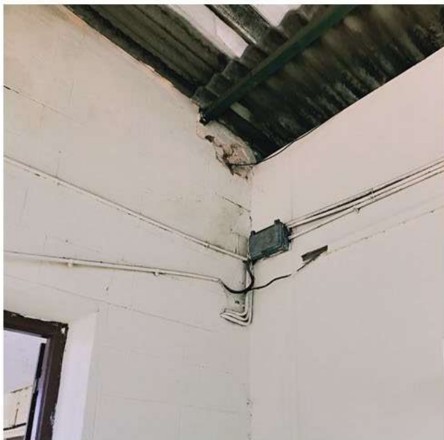
Figure 21: Error in use of new material – Thiruvananthapuram Railway Station replacement with incompatible material -- Shimla Railway Station
