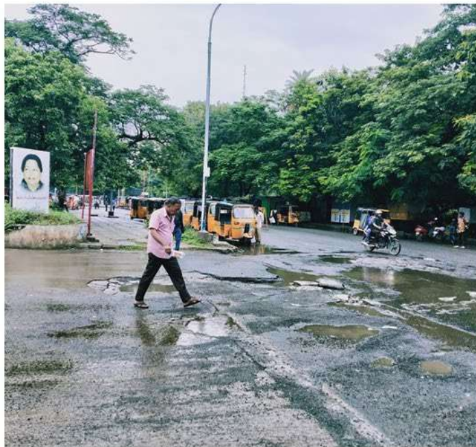
Figure 32: Incorrect repair of road and laying of infrastructure -- leading to accumulation of water, garbage and causing inconvenience – Thiruvananthapuram Railway Station
