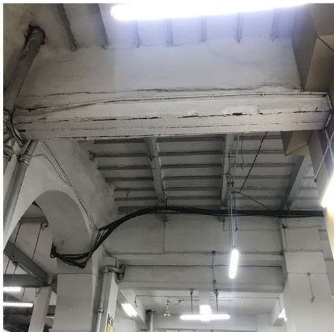
Figure 4: Deterioration of structural member due to excessive moisture percolation and incorrect repair -- Howrah Railway Station
