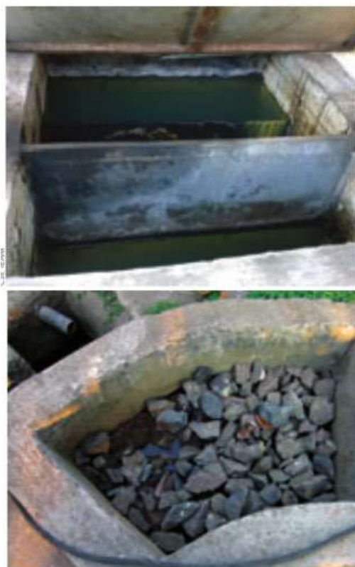
Figure 18: Phytoid based DWTS System (Photo Courtesy: CSE)
