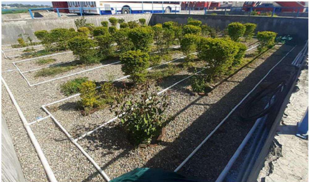
Figure 7: Executed SBT (200 KLD) at Jammu Airport, Jammu (Photo Courtesy: CSE)
