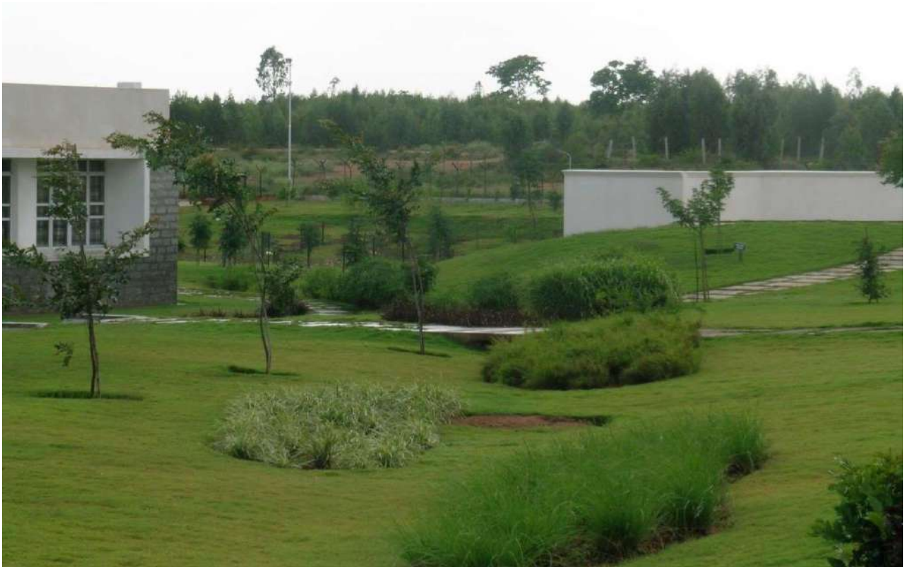
Figure 4: Photograph showing Swale (Photo Courtesy: InDe)
