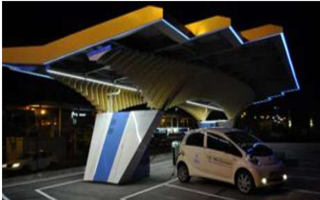
Figure 7-8: SRTPV powered charging station
