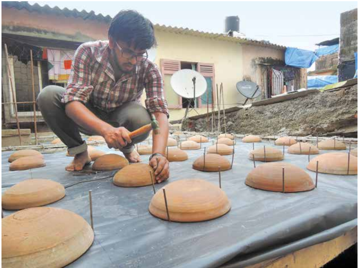
Low-cost material and innovative design can combine beautifully to improve thermal comfort and, thus, liveability of self-constructed houses
