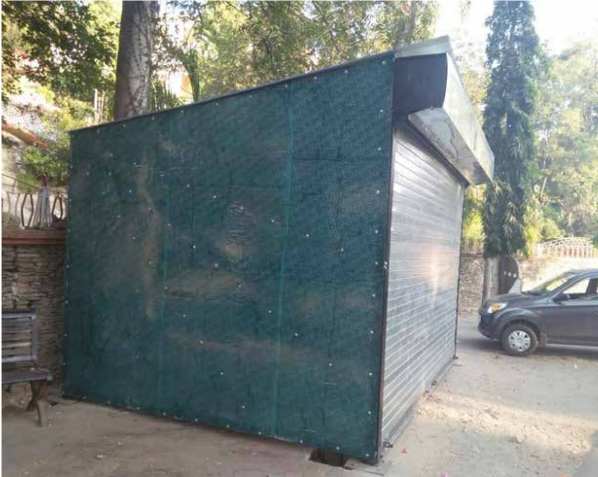
Newly constructed Docking stations at Aravali Vatika, Near Fateh Sagar Lake
