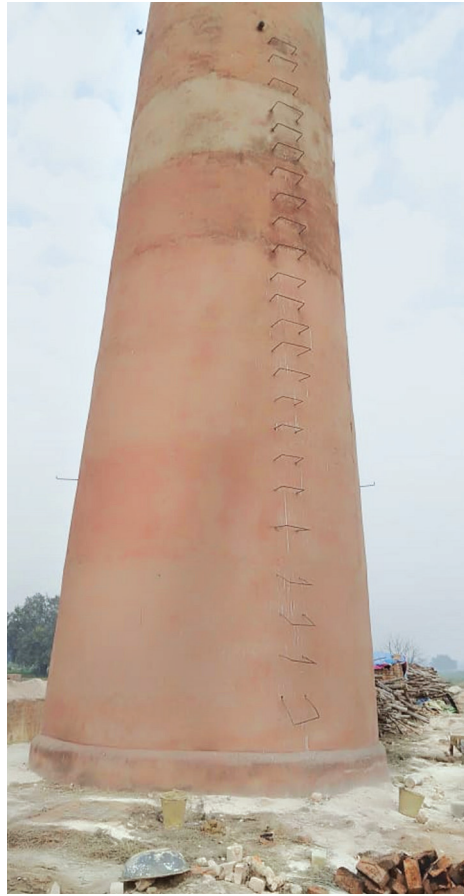
Figure 2: Monkey ladder without platform. (Kanpur, UP; 21-Feb-2019)
