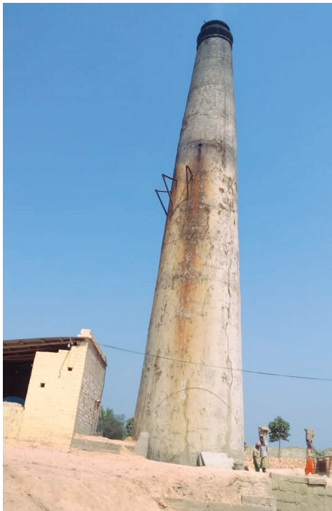
Figure 3: No ladder or platform (West Bengal, 09-Mar-2019)
