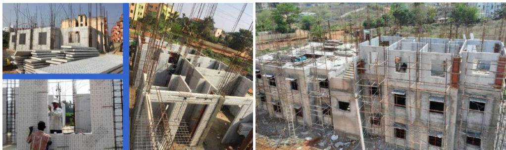
Figure 39: EPS technology for construction - Demonstration housing project by BMTPC at Bhubaneswar
